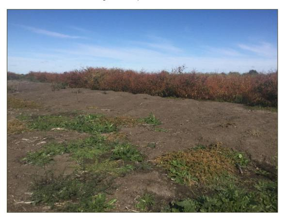
Figure 20: Excavated channel spoil prevent inundation to the east.
